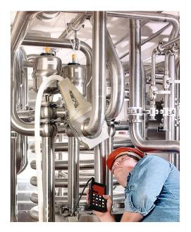
FIGURE 26.47 Stainless steel sanitary tubing joints should be made by automatical orbital welding where possible (Kopitzke et al., 2006).
