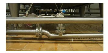
FIGURE 26.41 Non-drainable pipe (Hauser et al., 2007).
