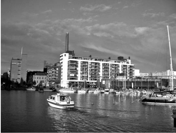
Plate 4.3 Waterfront development in Helsinki, Finland
