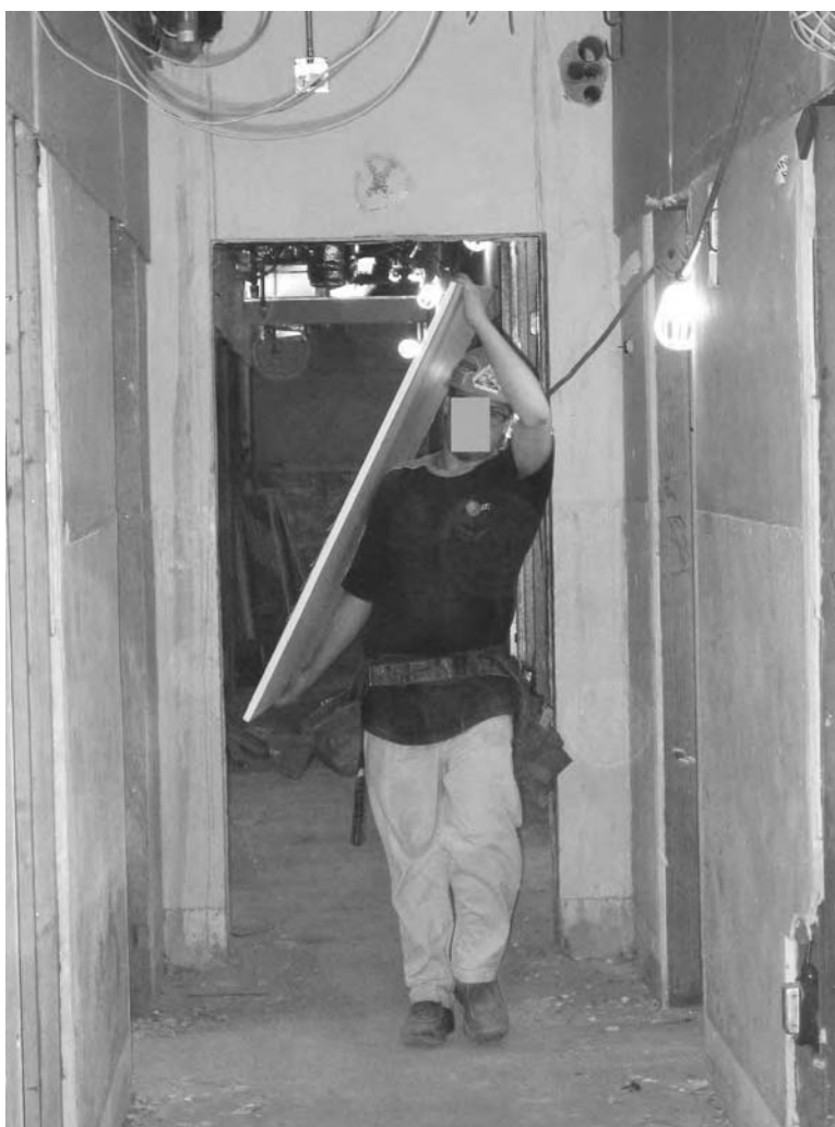
FIGURE 50.8 Worker manually handling drywall sheet.
