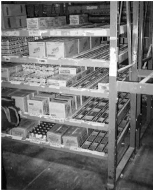
FIGURE 45.15 Gravity-fed flow racks.
