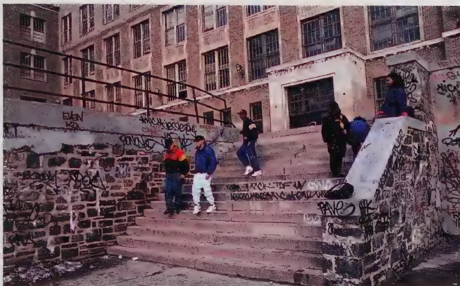
Century-old inner-city schools are sad examples of the decaying infrastructure.
