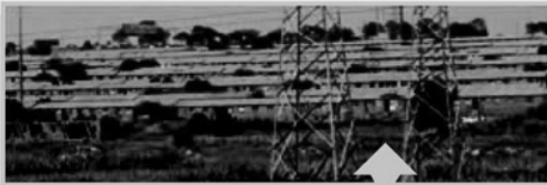
Former hostels in Soweto
