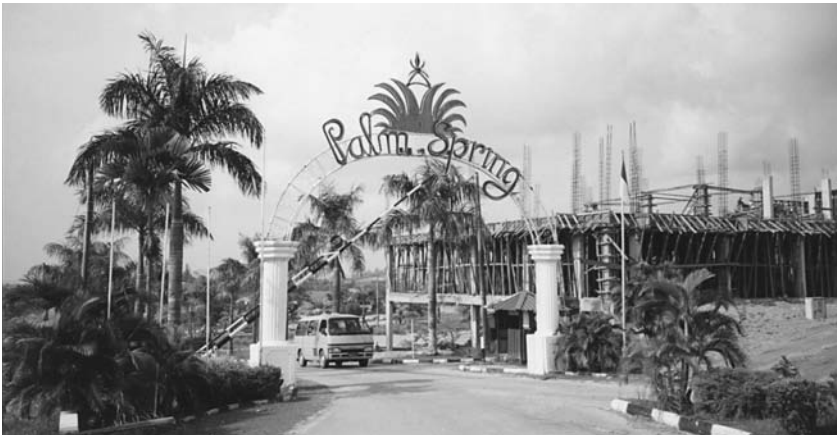
Entrance to the half-finished housing estate Palm Spring. Photo by author.
