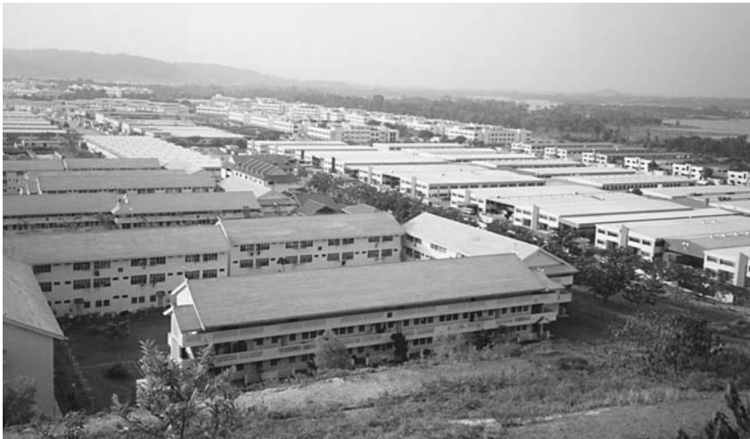
The Batamindo Industrial Park. Photo by author.
