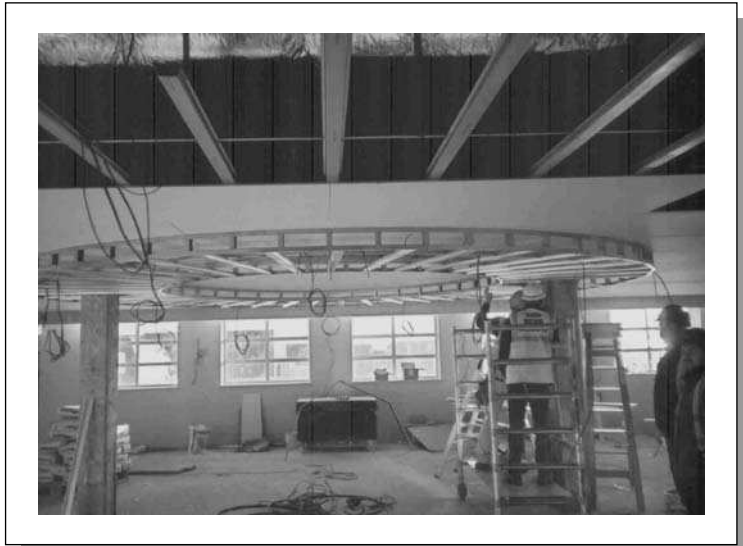
Illustration 9.3 Interior fitting out in progress
