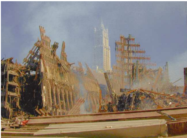
Figure 18.9 View of the World Trade Center after collapse. Note the exterior outer support columns, which are about the only structural components still standing. (Courtesy of Michael Rieger, Federal Emergency Management Agency, Washington, DC.)
