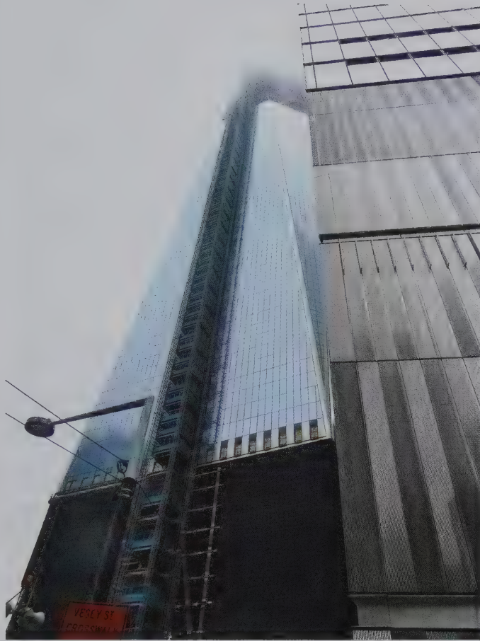
Freedom Tower under construction at the World Trade Center site in New York City. The tower opened in 2014. It stands 1,776 feet tall and will be surrounded by several other buildings, and a memorial to the nearly 3,000 people who were killed in the terrorist attacks that demolished the Twin Towers in 2001. How did those attacks change the American justice system?
