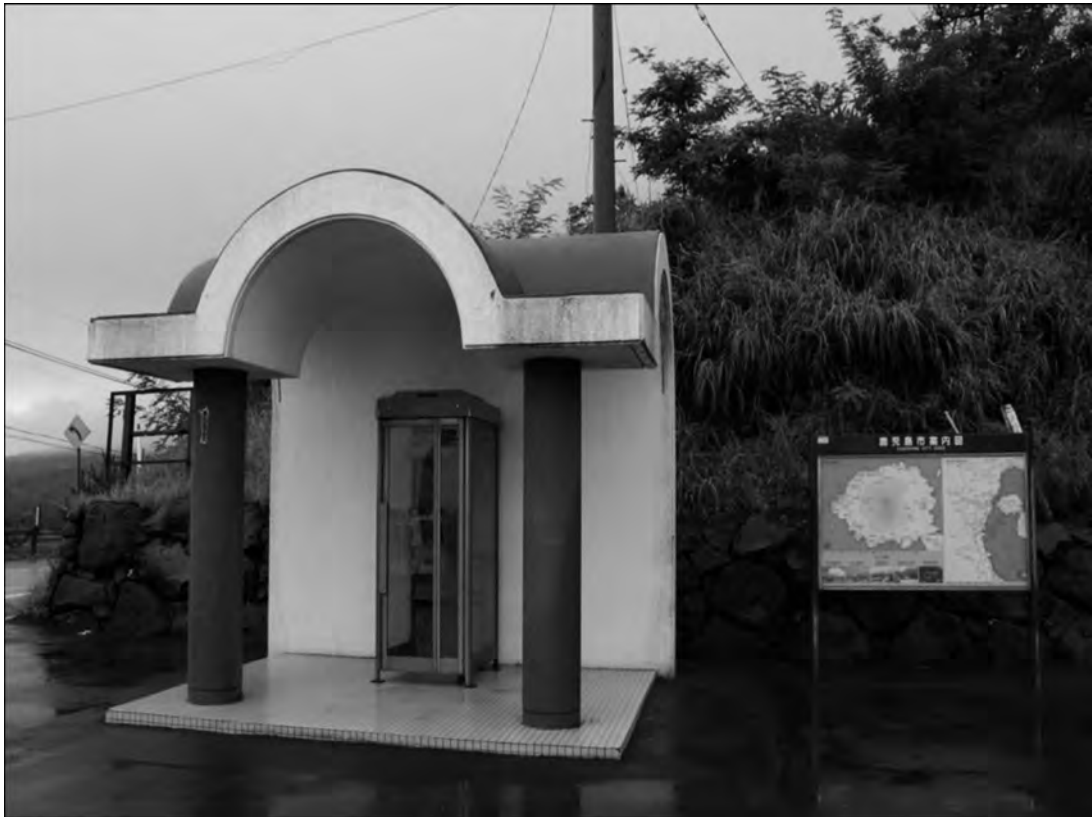
Figure 9.7 Public phone on Sakurajima Island with a concrete roof to protect against ashfall and more serious eruption fallout
