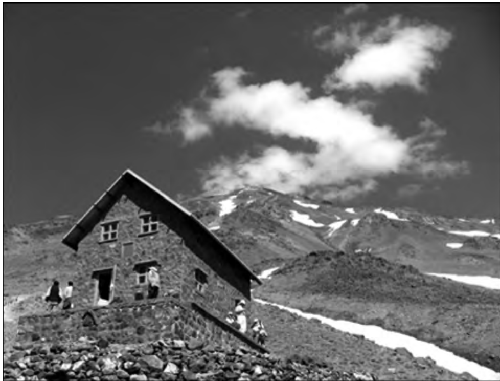
Figure 12.5 Simorgh camp, Mt Damavand 4150m, south-west route
