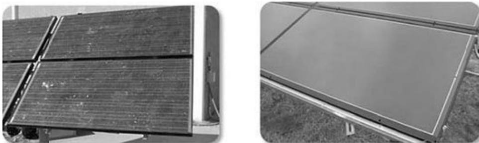
Fig. 16.4. Examples of multi- crystalline modules (left) and amorphous – silicon thin film modules (right)
