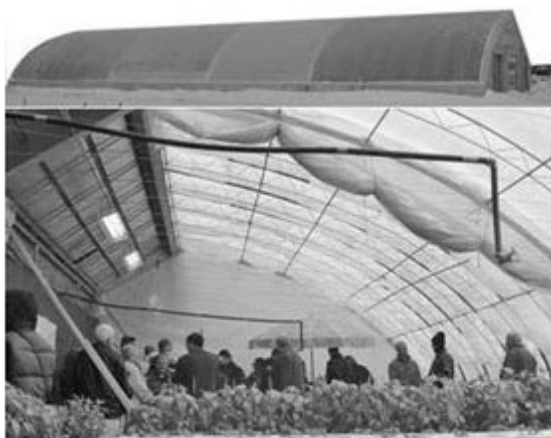
Fig. 16.12. Solar powered greenhouse heating.
