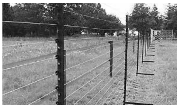
Fig. 16.6. Solar powered electric fence
