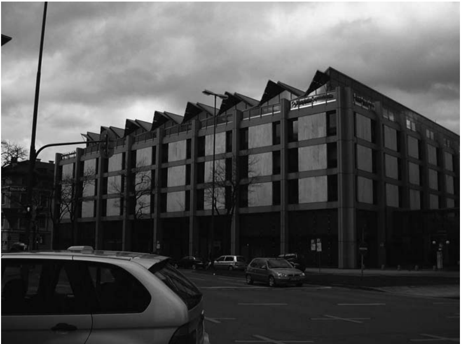
Figure 6.3 Bayerische Gemeindebank (Former Site of the Wittlesbacher Palais)
