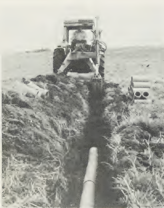
Fig. 22.4 Trenching with multi-purpose machine. The swivel post is being used in the fully offset position to aid the operator's view of the work. (McConnel)
