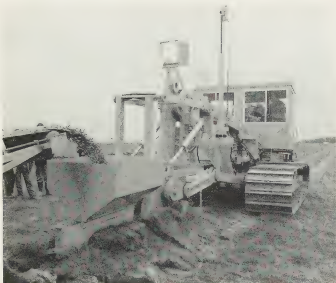
Fig. 22.10 Plough trencher equipped for laying plastic drainage pipe with gravel fill. The V-10 air-cooled diesel 275 hp engine employs independent hydrostatic drive to oscillating tracks. Single leg parallelogram mounting and laser depth control. ( Mastenbroek 25-20 Plow )
