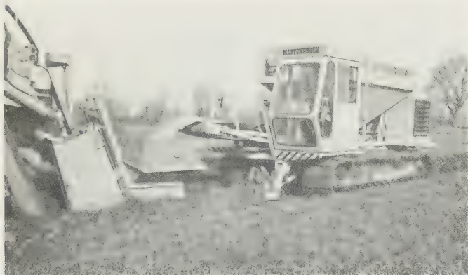
Fig. 22.6 Contractor's self-propelled gravel truck working in a growing crop in the same tracks as the medium-powered (145 hp) chain trencher-pipelayer, providing gravel fill and back-filling with staggered blades in a single bout to minimise crop damage ( Mastenbroek )
