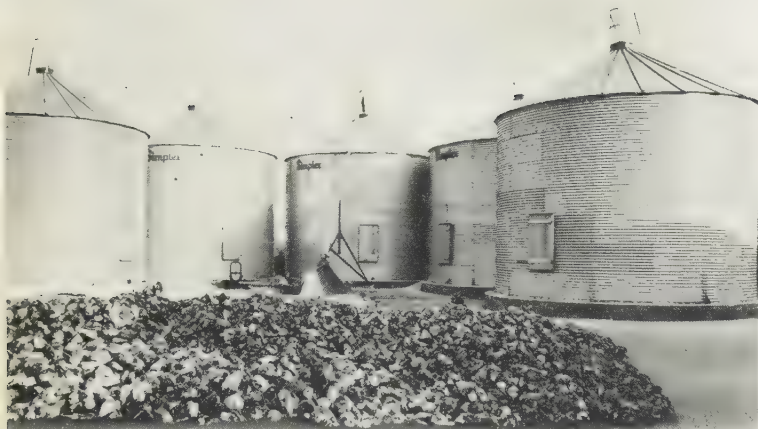
Fig. 18.15 Group of cylindrical outdoor ventilated bins with central filling and emptying by mobile augers.
