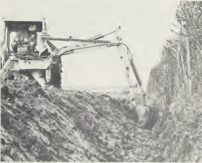
Fig. 22.2 Ditching with multi-purpose hydraulically powered tractor-mounted machine. (McConnel)
