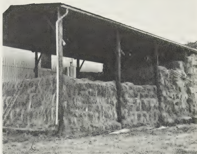
Fig. 18.4 A cheap building being used for a 'Dutch' hay-drying system. The fans are suspended from a rail so that they can be raised as filling proceeds, and to provide for movement from one bay to another. ( Electricity Council )
