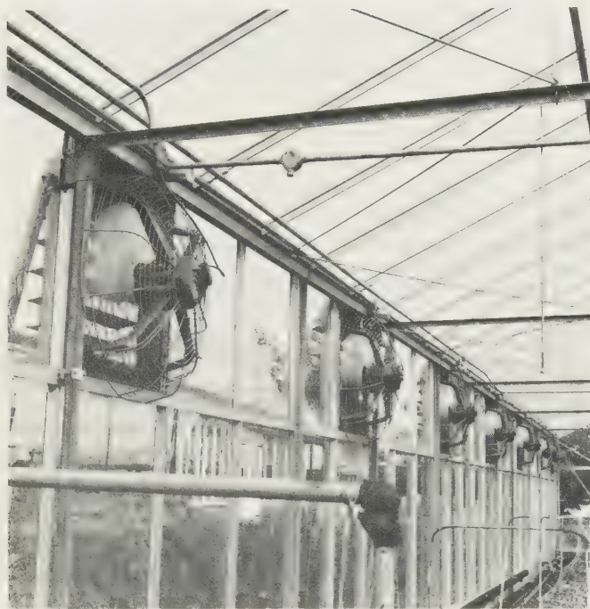
Fig. 23.10 A series of 0.6 m (24 in) extractor fans in a block of Venlo glasshouses. ( Electricity Council )
