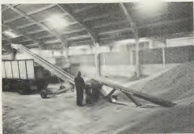
Fig. 18.25 Grain collector with endless rubber belt and flaps coupled to endless-belt elevator for lorry loading. The collector incorporates hydraulic-powered elevation and slewing, and is able to work effectively where well designed above-floor ducts are used. (Fyson 'Alligator')
