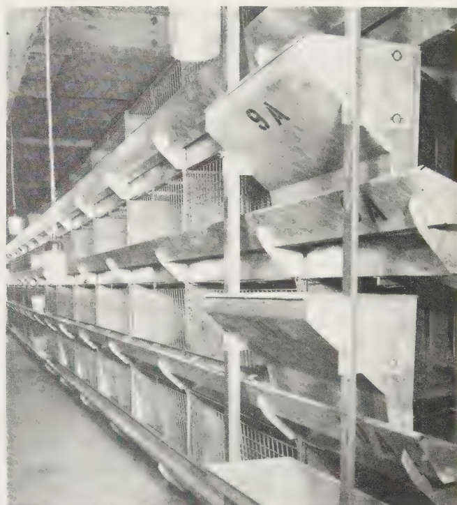
Fig. 23.18 Ventilation by perforated polythene duct (top left) in battery cage house. (Crown copyright photo)
