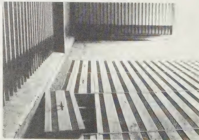
Fig. 18.17 Sectional multi-purpose drying floor of hardwood with inserts of perforated metal. (Challow)
