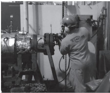
Figure 10. Vibratory tool disassembly the coke barrel (maintenance activity).
