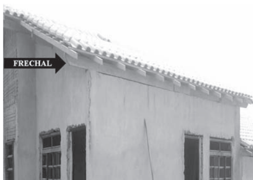
Figure 1. Setting of the main Roof Beam in a popular house.
