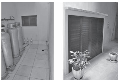
Figure 8. Floor drain close to LPG central.
